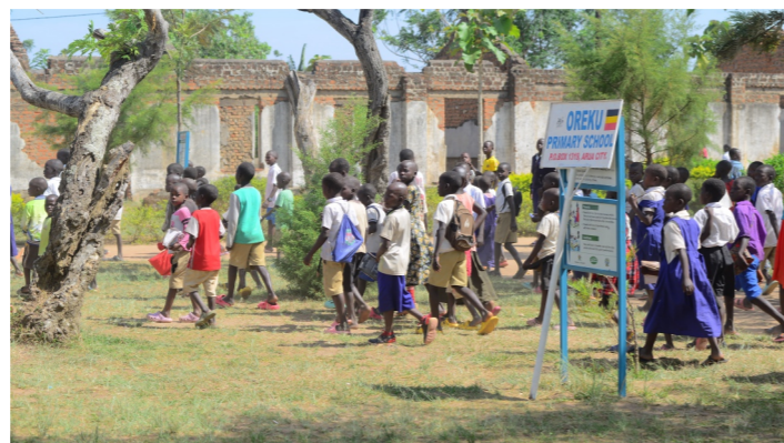
Pupils at Oreku Primary School in Arua walk past an abandoned and incomplete classroom structure. This is one of the classroom blocks being renovated by NSSF to create a better learning environment for the students
