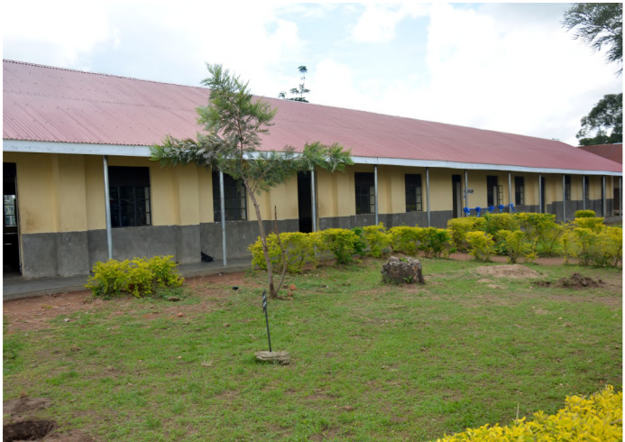
After renovation: The refurbished classroom block at Oreku Primary School in Arua, made possible through proceeds from the NSSF Kampala Hills Run
